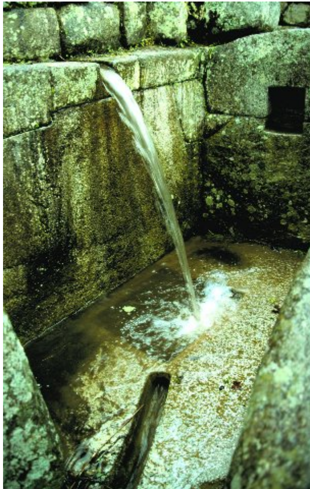
The water supply canal ends in a series of 16 semiprivate fountains, the first of which was for the use of the Inca emperor Pachacuti.
