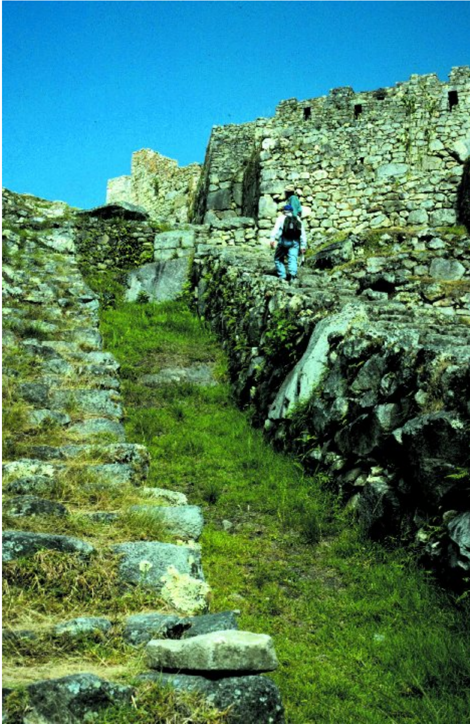
The primary component of Machu Picchu's drainage system is the main drain, which divides the agricultural and urban sectors of the city.
